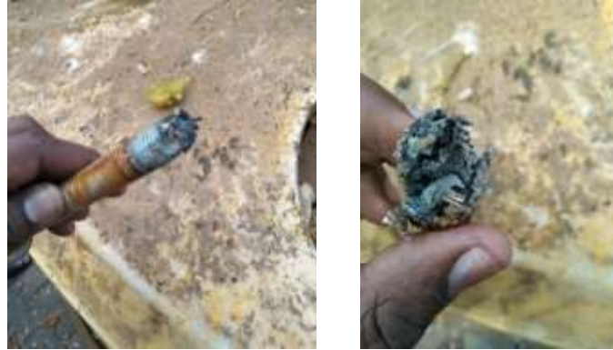
BD09 Failed Bolt
