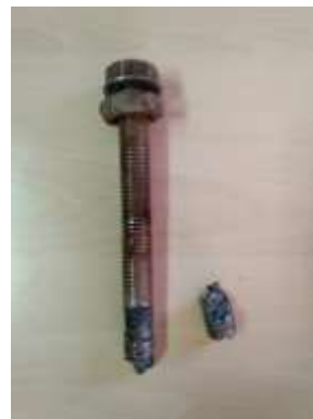
BD08 Failed Bolt
